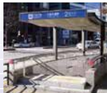
▲An entrance / exit for a subway station
