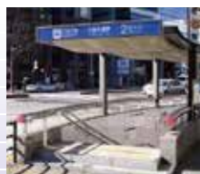
▲ An entrance / exit for a subway station
